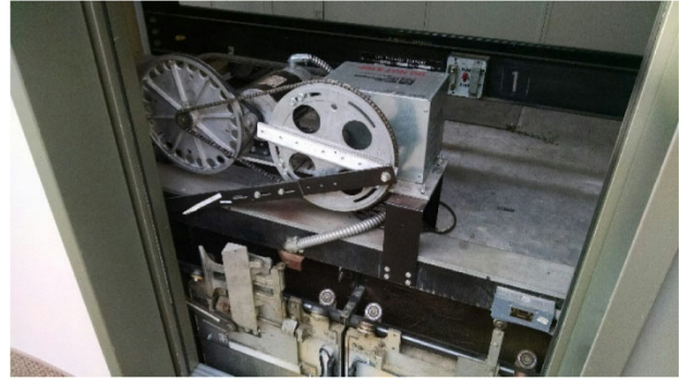
1990s Retrofit of a QL Operator on a Screw Operator Tubular Track Car Front (w/ original hanger, clutch & track)
