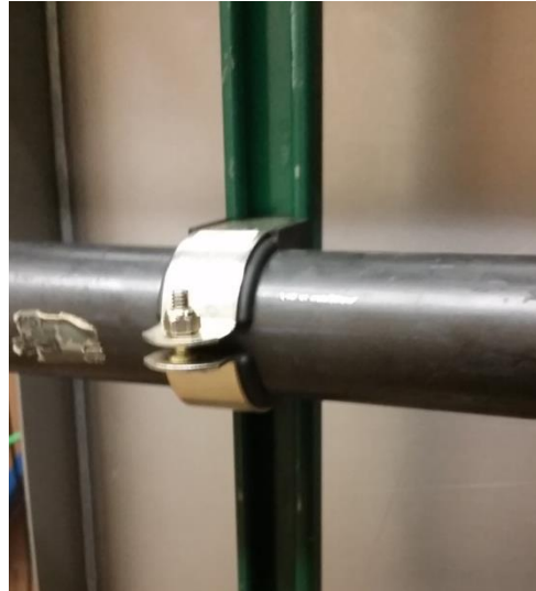
Figure 15: Pipe Stand Isolation Installed
